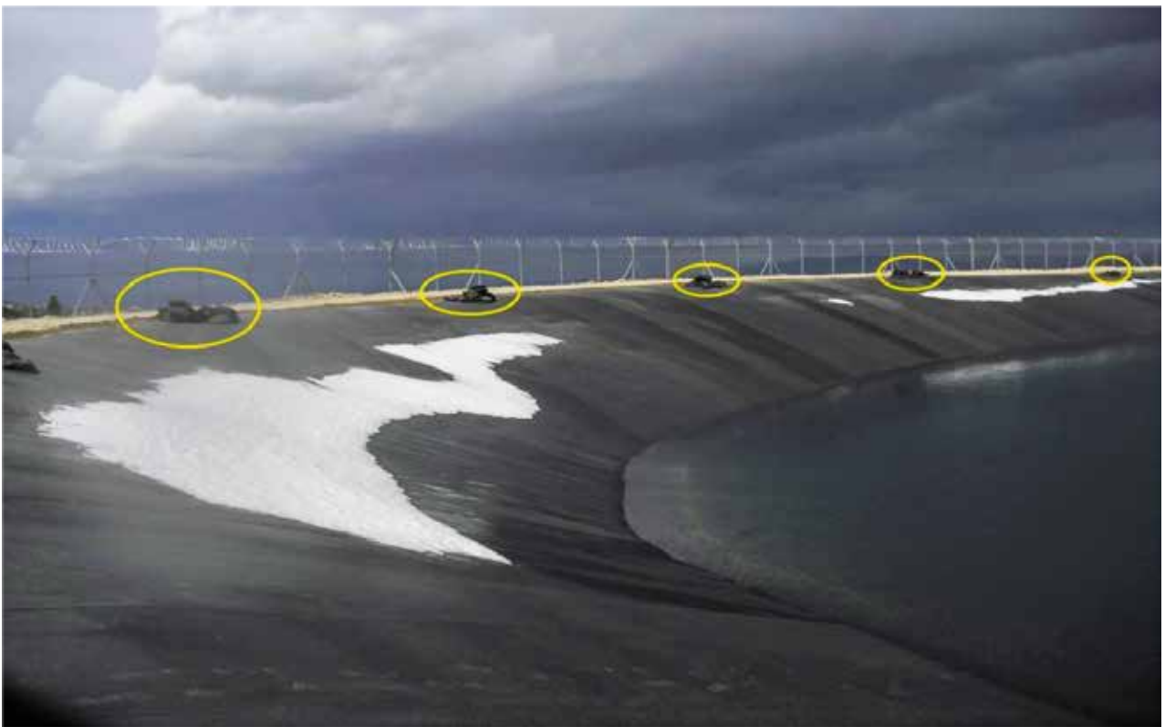
Membrane on the empty pond surface may swallow and tear off due to wind effect. EPDM sand bags are prepared in order to prevent this effect. EPDM sand bags, which are prepared to be placed on the surface of the pond to be drained, are kept on the top elevation of the pond at certain intervals.
