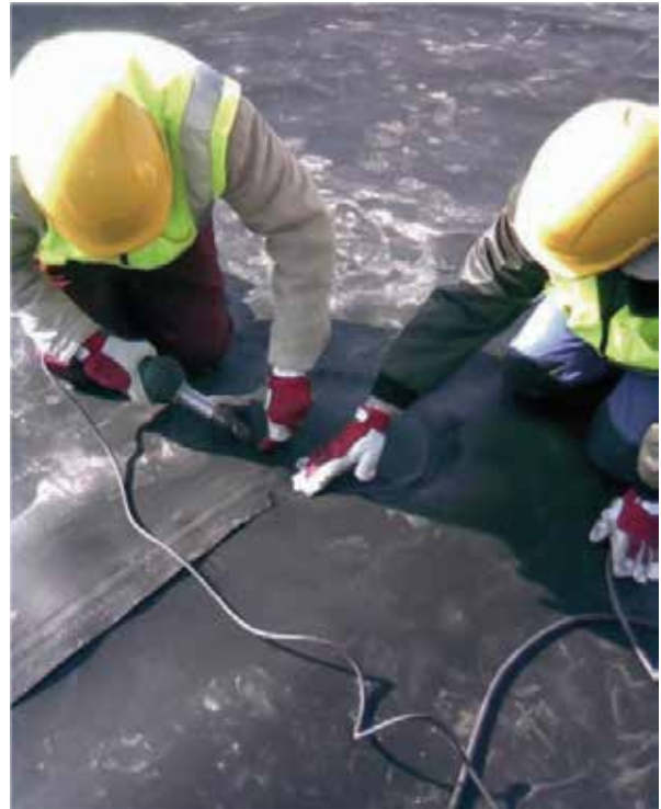
Areas, which require repair, are repaired easily.
