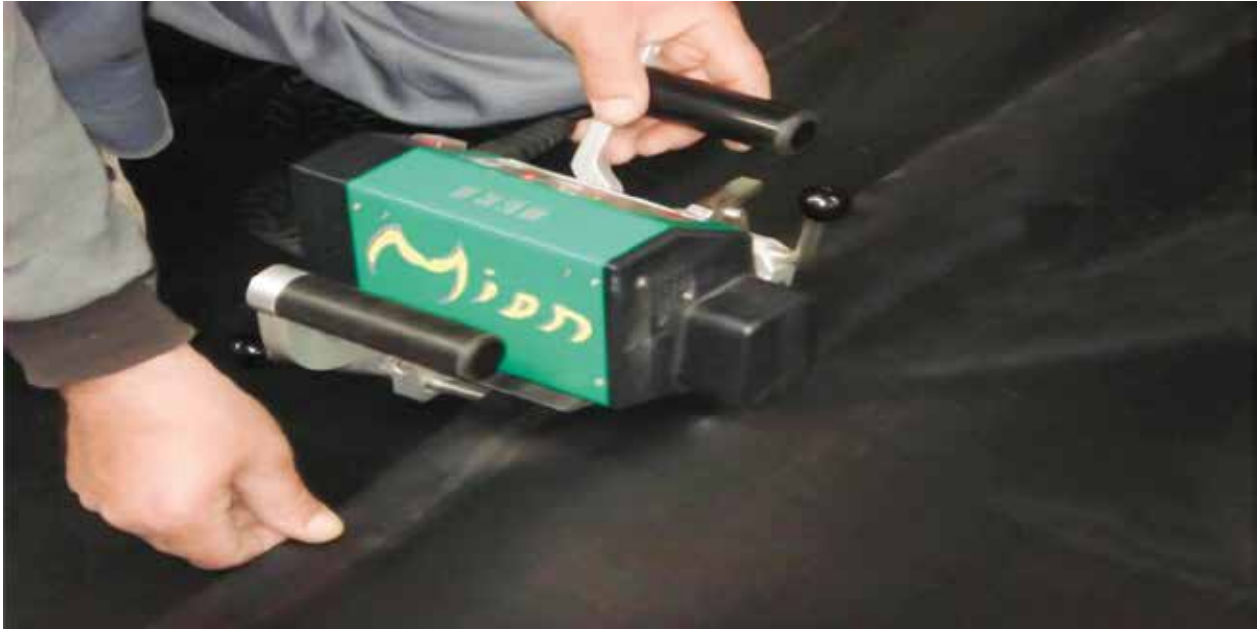
Welding with automatic welding robot
