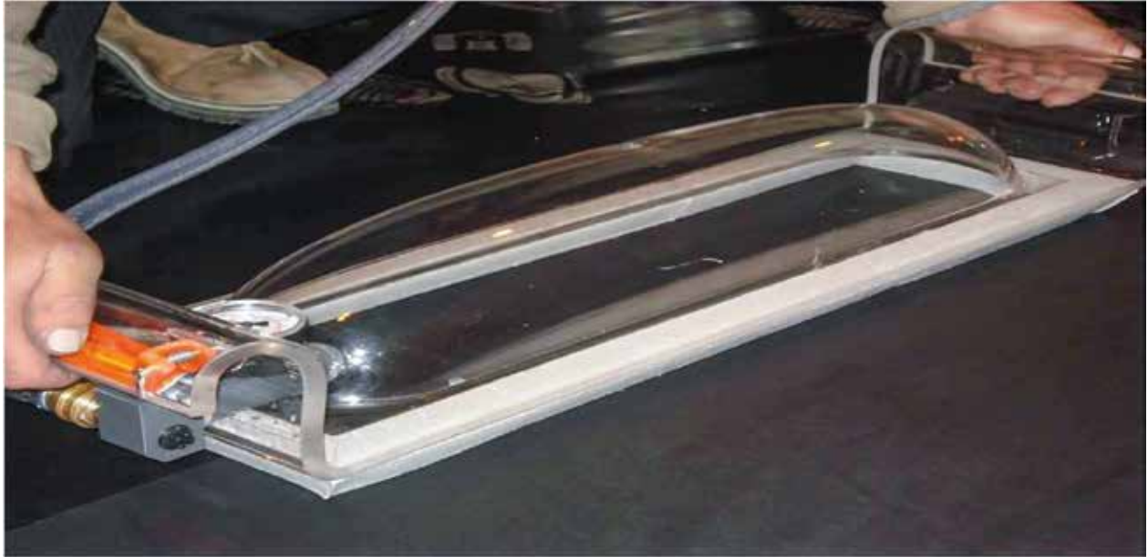
Welding control with vacuum test device
