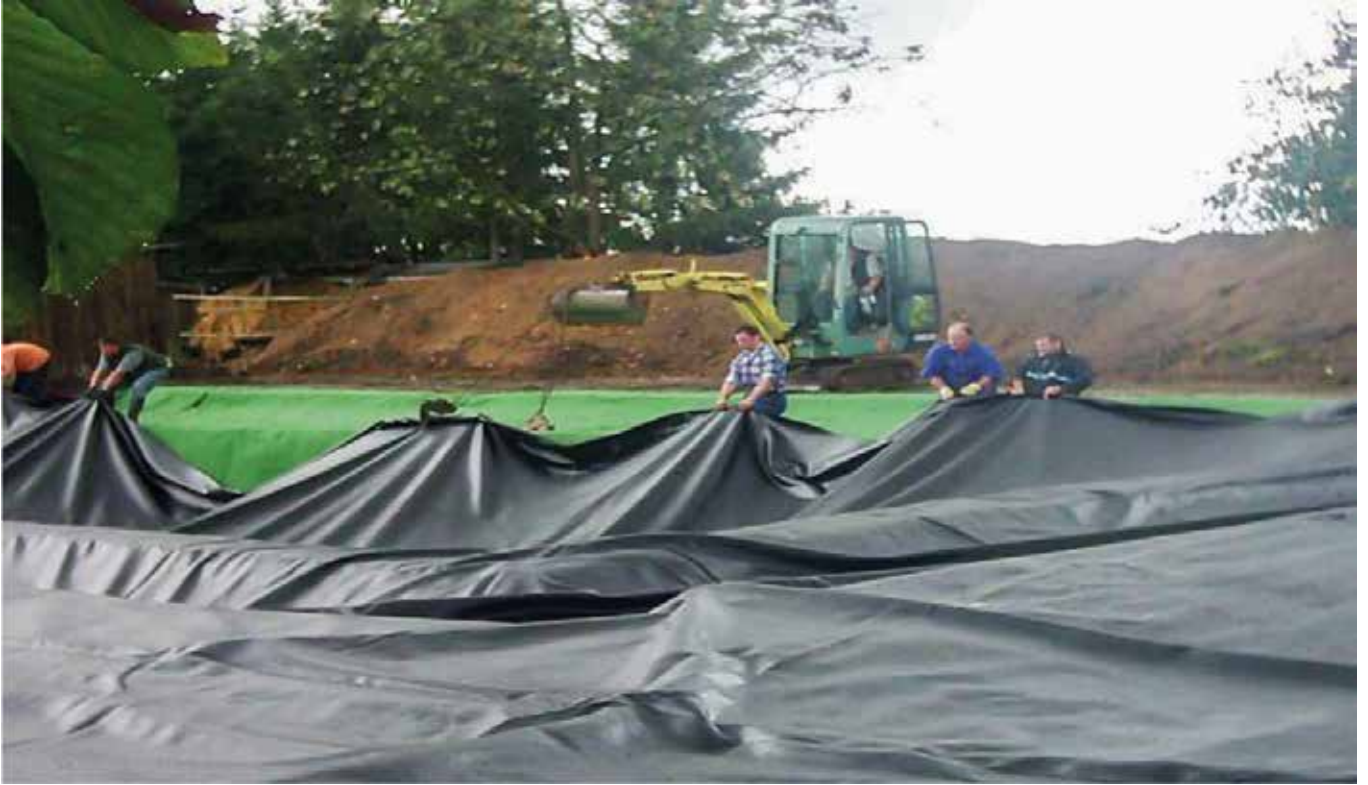
Laying of the large panel prepared in accordance with pond project
